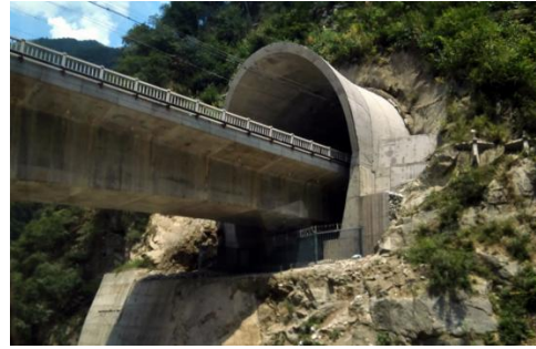
4.3-6 倒削竹式洞门
