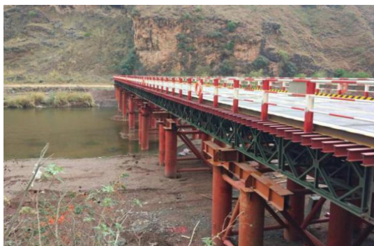
12.2-11 施工便桥便桥护栏
